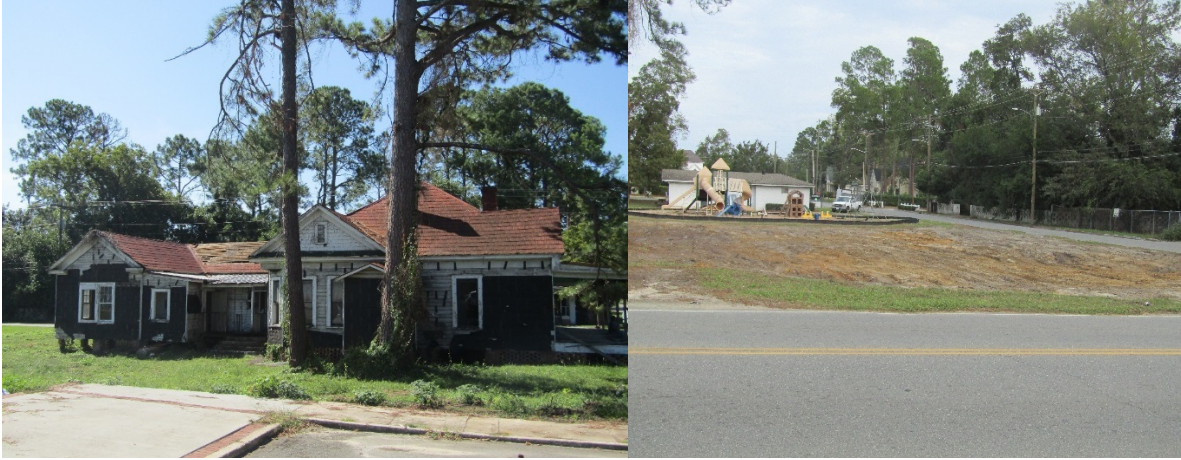
Figure 25: Property on South Scott Street that is severely damaged before and after demolition
