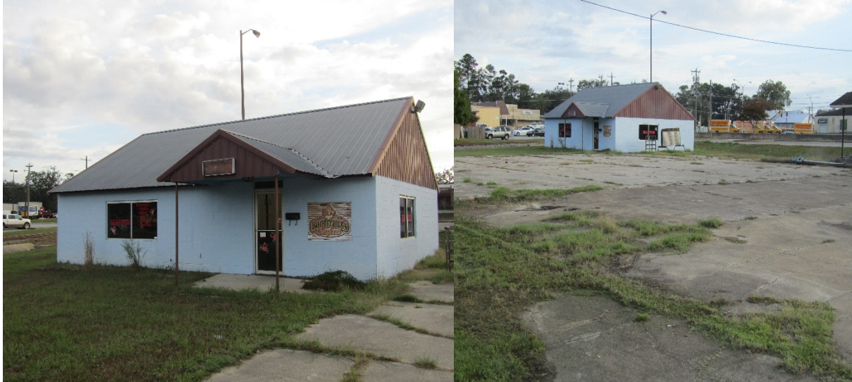
Figure 44: Unoccupied building on South Butler Street with a land space.
