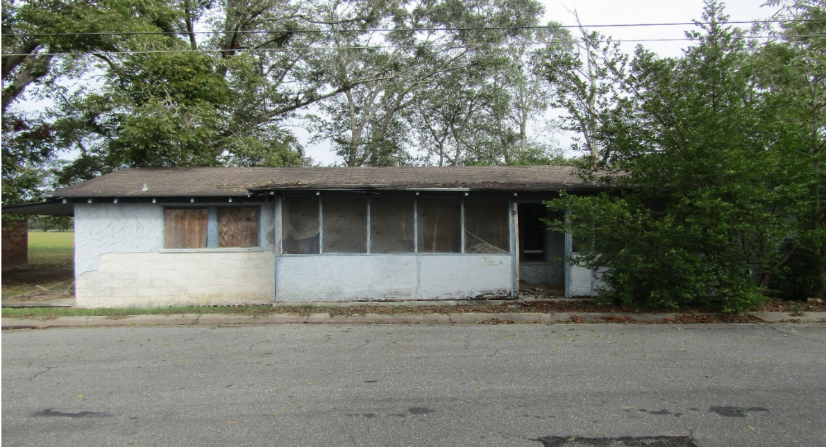
Figure 33: Abandoned building on Robinson Street
