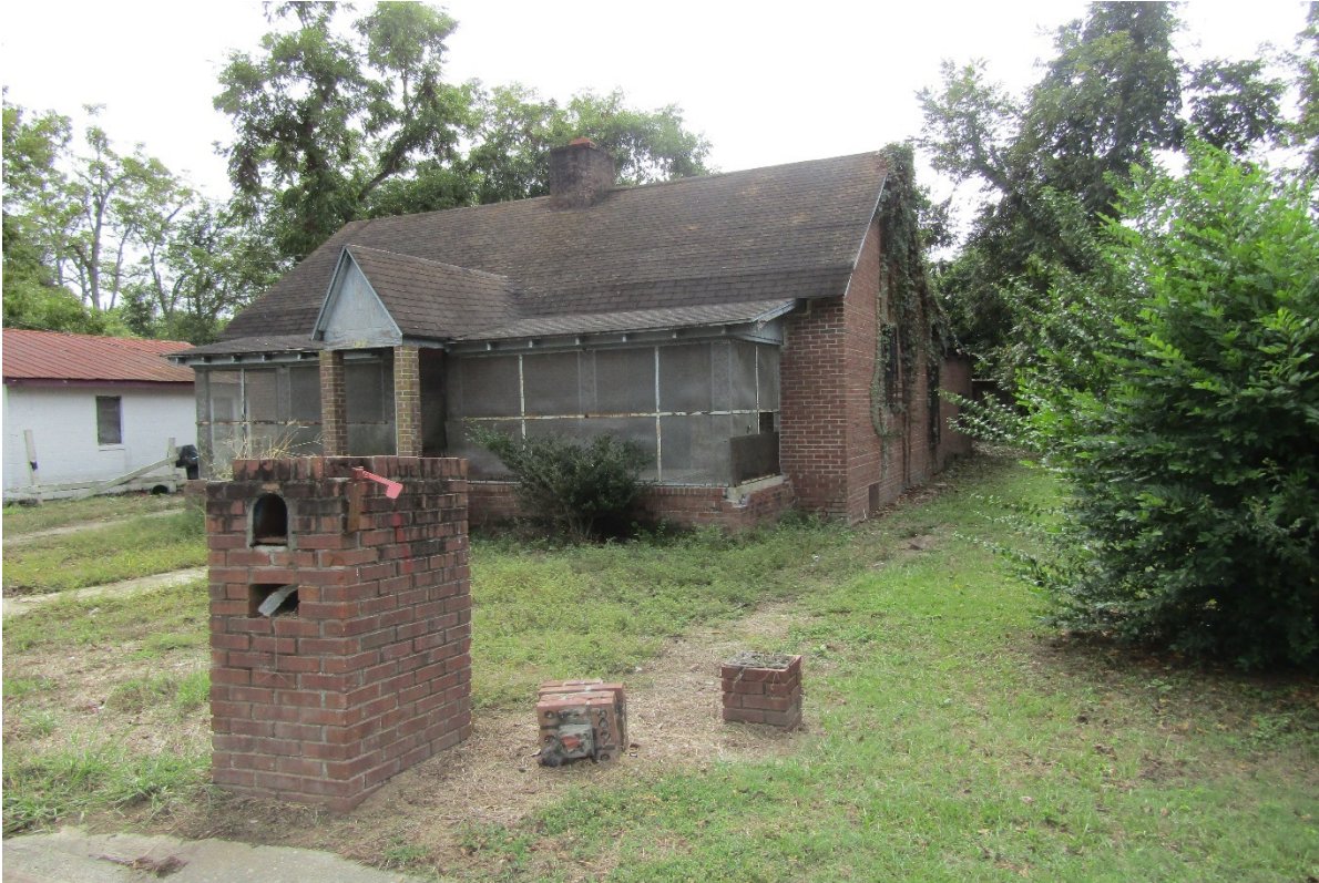
Figure 34: Substandard vacant building on Robinson Street
