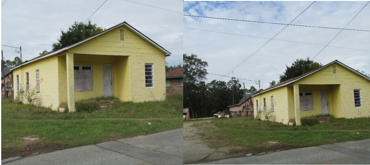
Figure 32: Substandard vacant building on Ellis Street
