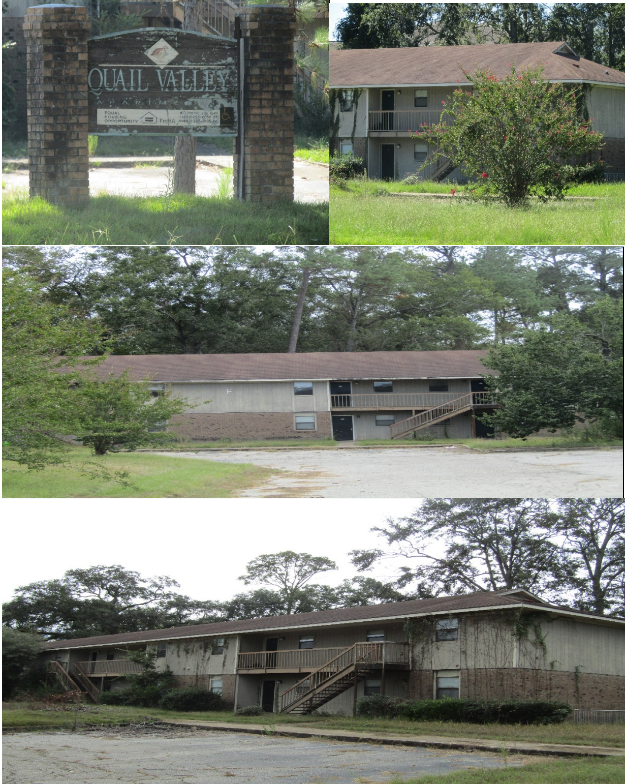
Figure 28: A Multi-Unit Apartments on Highway 19 that needs complete renovation which could be turned to Extended Stay Inn
