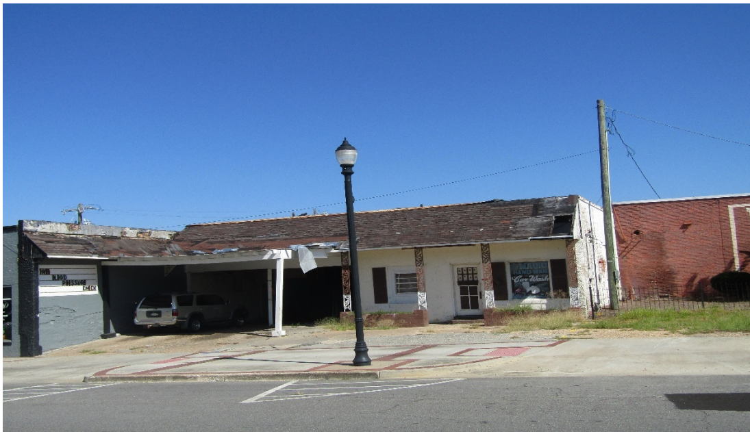
Figure 24: Property on East Broad street that needs renovation
