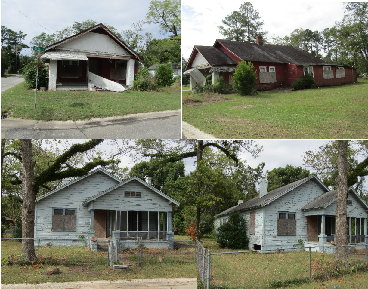
Figure 37: substandard buildings on Dyer Street
