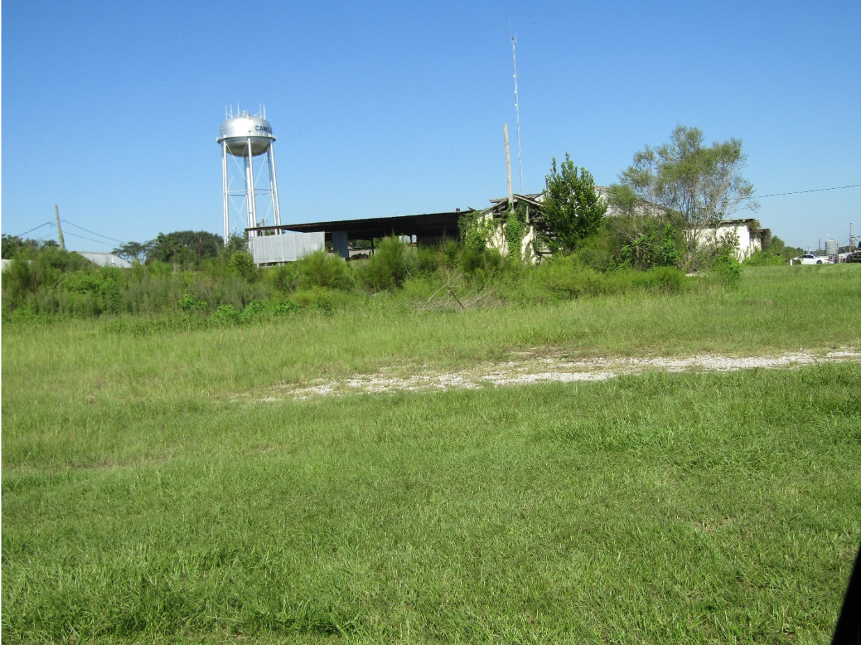
Figure 21: Vacant Parcel beside the abandoned building covered with leaves ( Development Potential)
